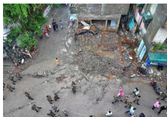
Remains of the day: Residents and security personnel at the site of the building collapse in Rohini's Sector 16 on Thursday. PTI
