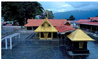
The court was considering queries raised by the Audit department on a contract to supply 1,000 cots for Sannidhanam staff. FILE PHOTO
