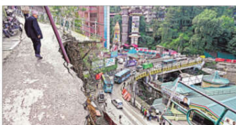
A damaged road is seen near a landslide site following overnight rainfall, in Shilma on Sunday. PTI
