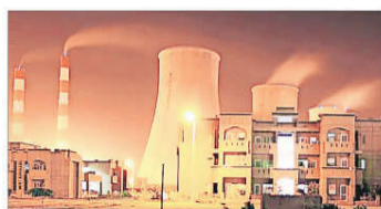
Thermal power stations are expected to take preventive maintenance to minimise forced and partial outages. REUTERS
